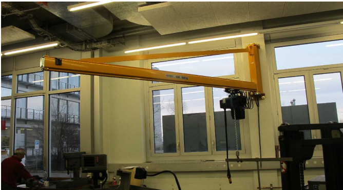
FIG. 17.1 – Installation of the wall crane in the student workshop.
