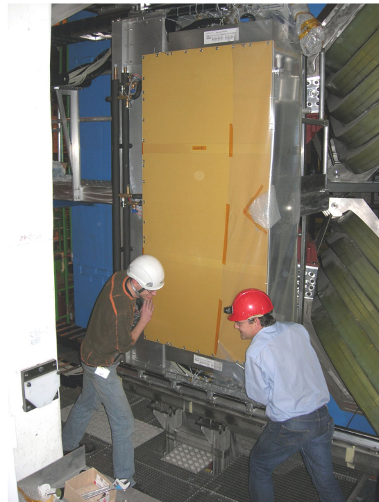
Figure 14.3: Installation of the LHCb TT-station at CERN.
